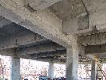
Concrete post and beam construction.
